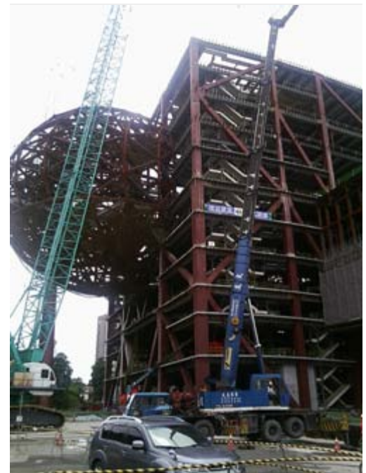
Taipei Performing Arts Center construction site. In picture: the spherical Proscenium Playhouse
