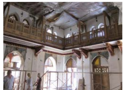
National Theatre Lobby under reconstruction
