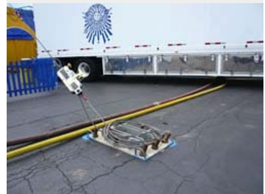
One of 50 tie-down plates anchored to the ground
